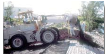
Cellular blankets provide an aesthetic alternative to poured concrete walls and other armored installations
