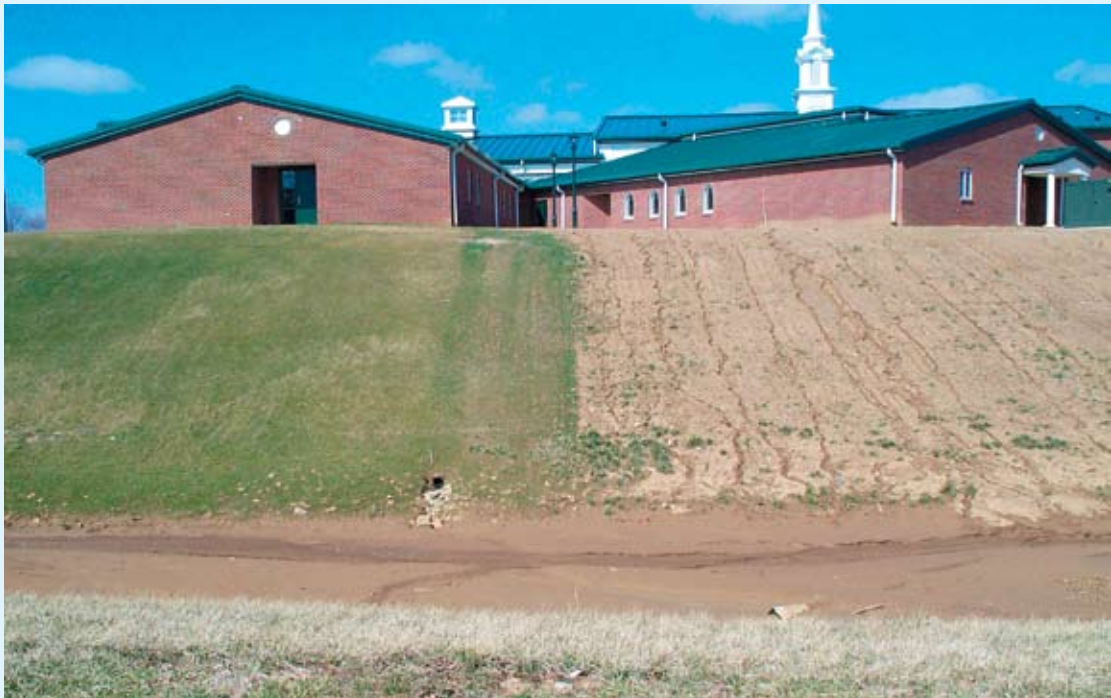
The value of seed on a slope: the left (seeded) section shows almost no erosion; right side rills are quickly becoming gullies. Seed and mulch slopes as soon as final grade is established for best results. Bare areas must be seeded or mulched within 14 days if no work is planned during the next week.
