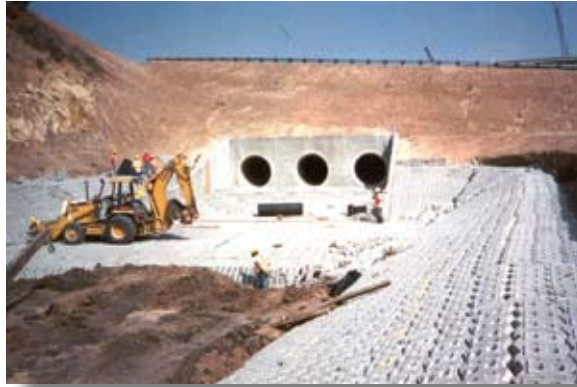
Concrete and plastic cellular blankets, like this open-celled concrete block product, provide heavy armoring while supporting vegetation that softens the final look.
