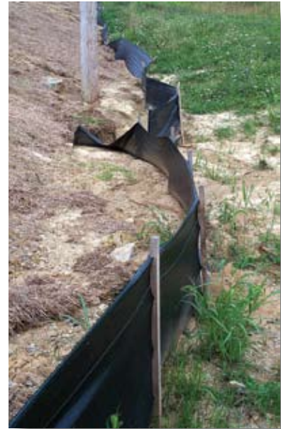
Silt fence is functioning well, but needs maintenance. Set fences back from the toe of the slope, to allow room for sediment to accumulate and maintenance.
